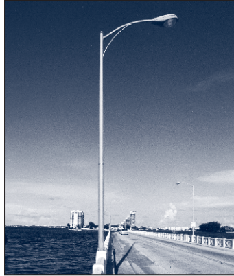
Venetian Causeway Miami, FL Installed Circa 1951
